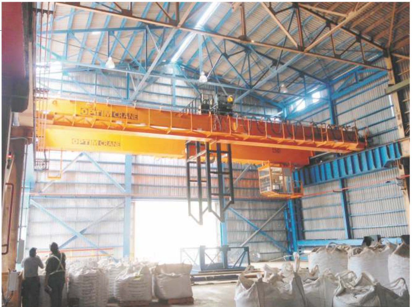
Special crane for transporting . Nickel Plant, Guatemala
